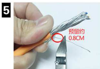
5 cut off ground wire, reserved 0.8 cm
